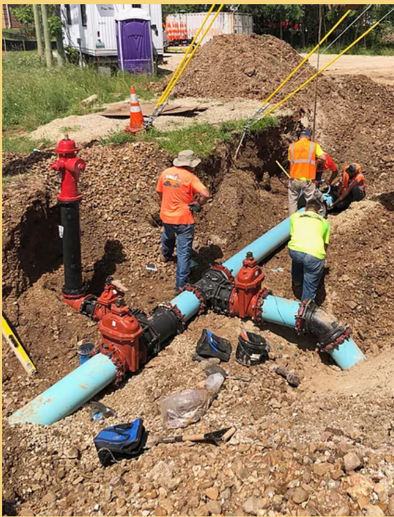
Workers with M&M Landscaping & Construction work on the main waterline being relocated as part of the MoDOT interchange project on Highway 54 near Mt. Carmel Baptist Church on Business 54.
