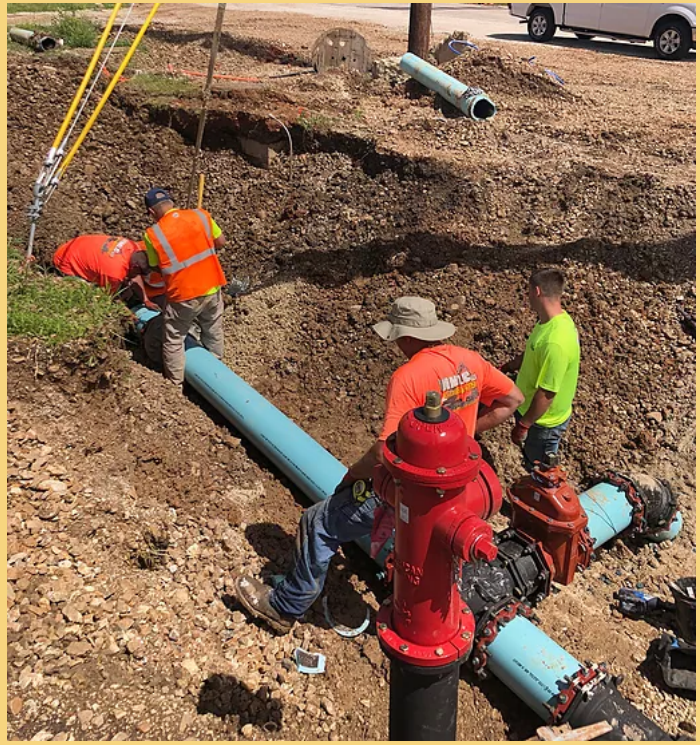
Workers with M&M Landscaping & Construction work on the main waterline being relocated as part of the MoDOT interchange project on Highway 54 near Mt. Carmel Baptist Church on Business 54.
