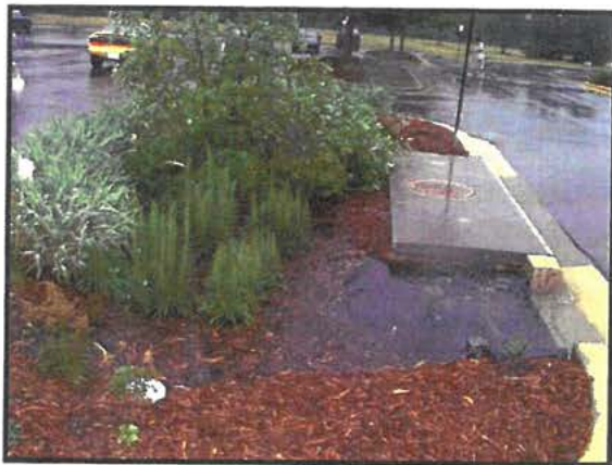
Bio-retention Cells: soil and plant-based filtration devices that remove pollutants through a variety of physical, biological, and chemical treatment processes
