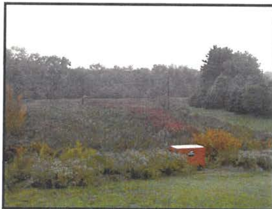
Storm water treatment wetlands are small constructed ecosystems that temporarily store storm water runoff and provide significant pollutant removal by sedimentation, adsorption, biodegradation, filtration and bioaccumulation.
